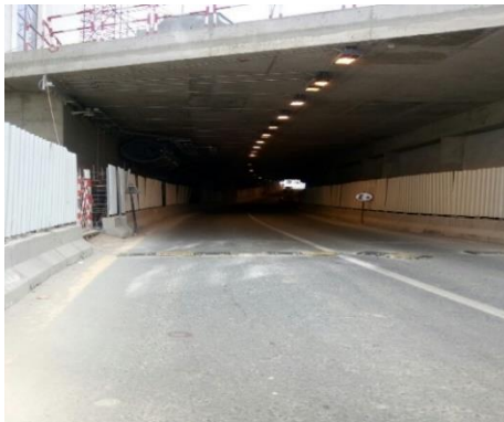
Fig. 4. Curved rectangular tunnel for cars, width = 9.2 m, length = 195 m and height = 5.8 m.
