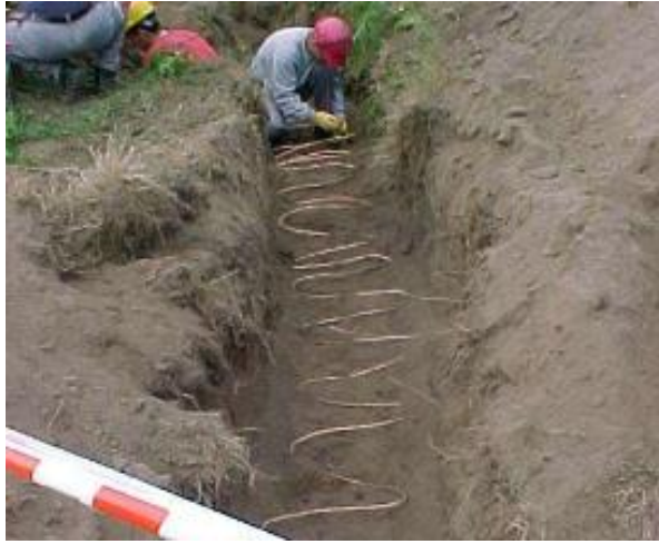
Fig. 1. Sinusoidal grounding electrode [13].
