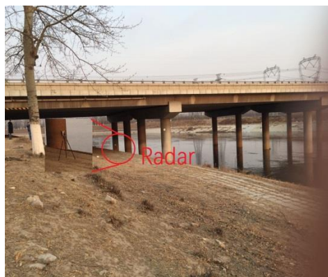
Fig. 3. Setup of the bridge vibration monitoring.
