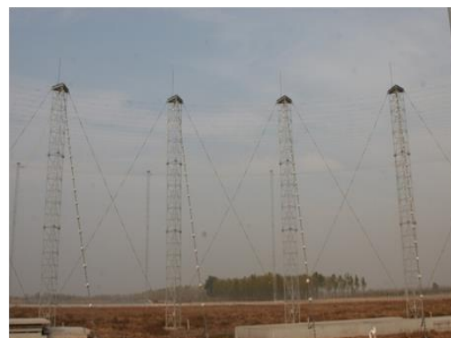
Fig. 12. The UCA-LPDA for direction finding.
