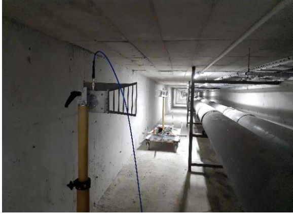
Fig. 5. Signal measurements and underground tunnel.
