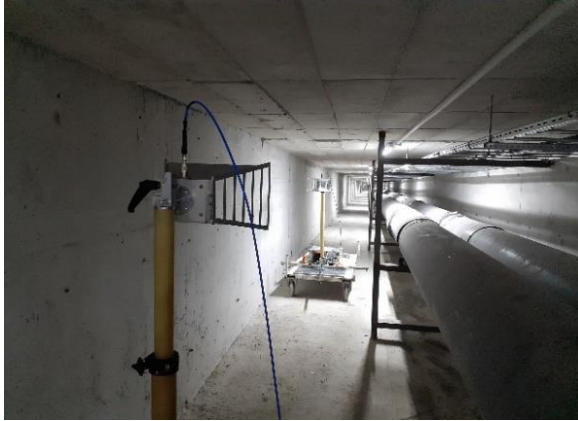
Fig. 5. Signal measurements and underground tunnel.
