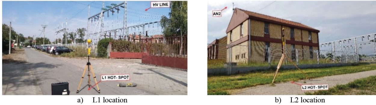
Fig. 2. Monitoring locations near the substation “Novi Sad 7”.
