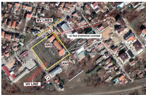
Fig. 1. Position of the substation “Novi Sad 7”.
